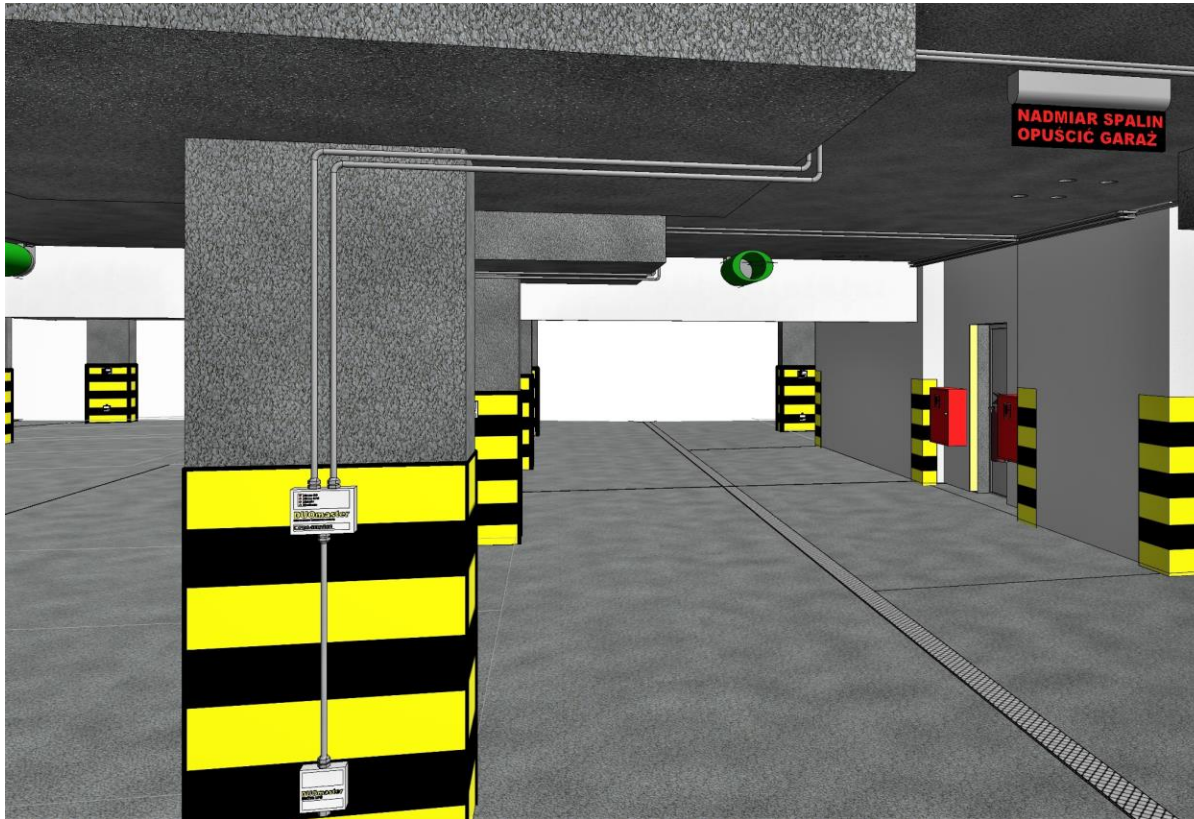
View of the garage with CO/LPG sensors and warning signs
